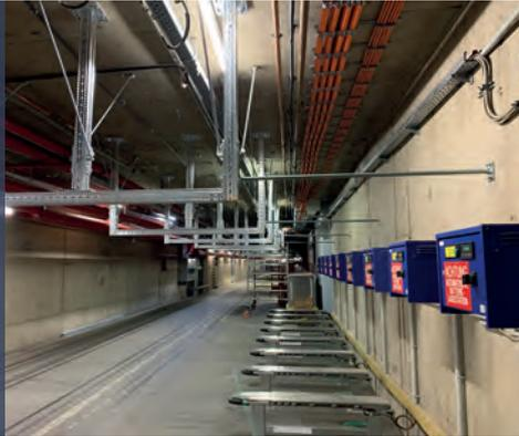
The geothermal ring pipeline is 1,500 m long, with nominal pipe sizes from DN 100 to DN 500 mm, and Sikla delivered more than 25,000 kg of material to secure it. The materials included 1,100 m of TP F 80 beam sections, 400 m of TP F 100 beam sections, 14,000 FLS F self-locking screws and 350 Simotec pipe shoes.
